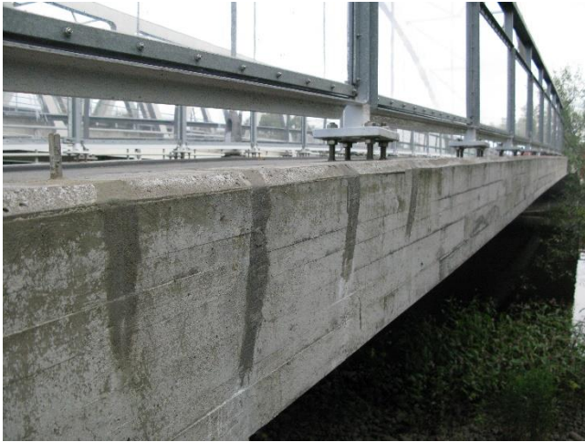
Figure 1. A bridge edge beam in Sweden with cracks that have been injected and sealed.
